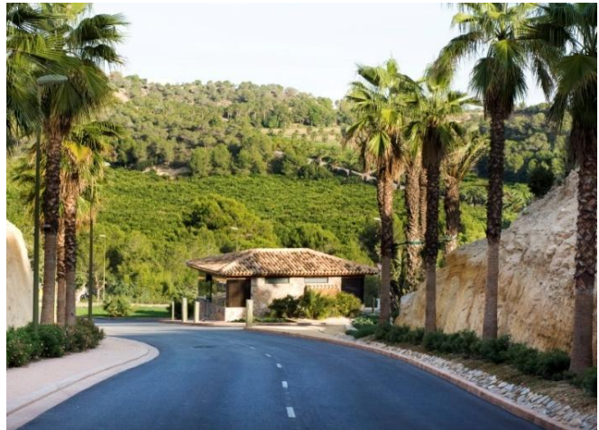
Entrance sign and the complex's security control.
